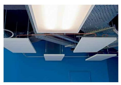
The form and surface of the heating and cooling sails were selected in such a way that they fit in perfectly with the overall architectural concept. Lighting elements were also integrated into some of the panels.
