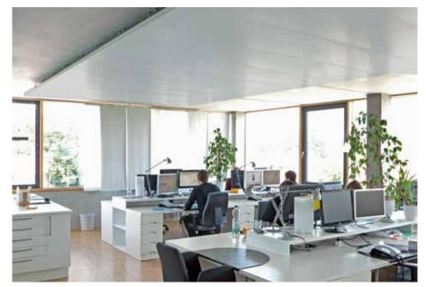
The climate in all of the office areas, including the cafeteria, is controlled with Zehnder heating and cooling ceiling sails. The lightweight panels made of natural graphite ensure particularly rapid, even and efficient temperature distribution.
