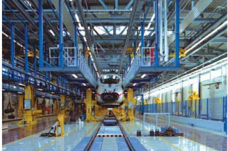
39 radiant panel modules were installed, with a length of 1,147 m. Placement of the panels required a large amount of skill in order not to be in the way of the crane rails running the entire length of the hall over the three sets of tracks.
