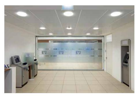
Comfortable indoor climate in the foyer: the Zehnder Carboline ceiling elements cool the space without so much as a sound or draught, and the lighting and air outlets harmonise with the cooling ceiling.
