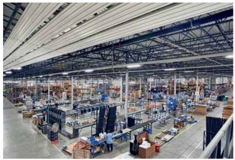
Zehnder ZIP radiant panels were used. An overall length of approximately 1,800 m was installed in 13,000 m<sup>2</sup> of plant area and 1,850 m<sup>2</sup> of office space, with ceilings ranging up to 30 m in height.
