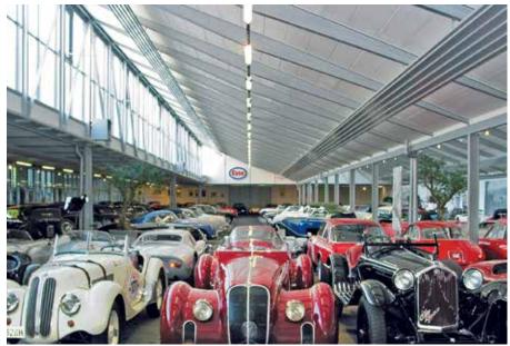
The showroom, which is located in a former factory, was equipped with radiant ceiling panels across the entire installation length of just under 400 m. This perfectly meets the particular climate requirements of a museum.
