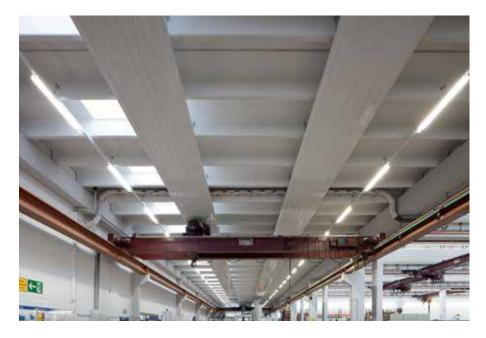
Even heat distribution in all areas of the hall: the radiant principle used in the ceiling panels means that the temperature throughout Reifenhäuser is draught free, comfortable and above all constant. As well as being pleasant for the workforce, this also helps the precision work at the machine components.
