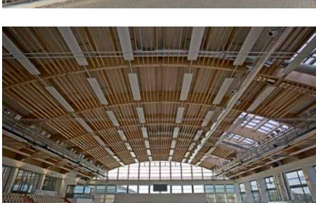
In order to heat the 5,000 m² large hall evenly and efficiently, the decision was made to choose Zehnder ZBN. A total of 372 m² of perforated radiant panels were installed on the wooden structure which supports the roof of the hall in order to absorb the sound.
