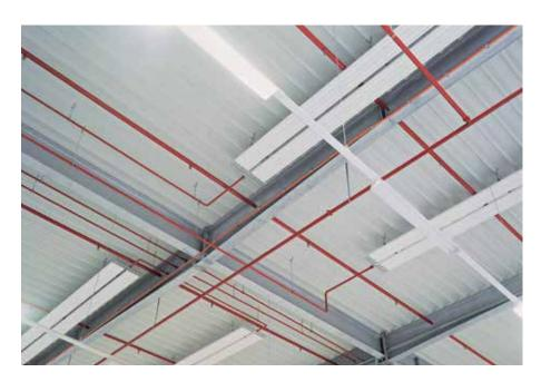
A total of 266 individual modules with a total length of 2,628 m were mounted. The great advantage: the panels no longer need to be welded, but can now be pressed or screwed into place instead.
