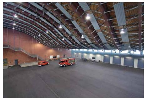
The floor space of the fire services training hall covers over 2,370 m². The increased energy efficiency of the radiant panels compared against air heaters has an extremely positive impact on operating costs.
