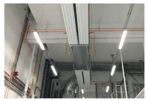
At Rubin Mühle Vogtland, ten Zehnder ZIP radiant ceiling panels, each three metres in length, were installed. This intelligent form of heat supply can be mounted approx. two metres below the hall ceiling in a flexible and customised manner.
