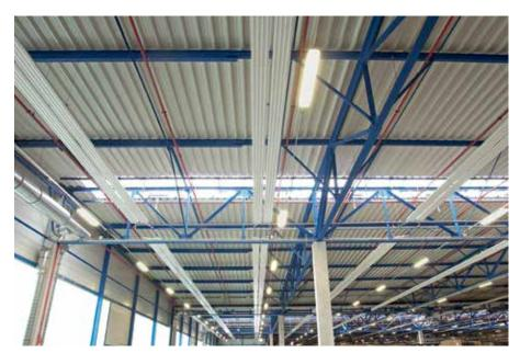
Emphasis is also placed on performance and efficiency in the area of air-conditioning technology, in the form of a Zehnder heating and cooling ceiling system. 20 km of Zehnder ZIP radiant ceiling panels were installed.
