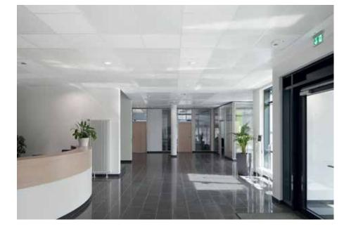
Among other areas, the heating and cooling ceiling systems were installed in all of RAFI Eltec's open-plan offices. The ceiling modules were installed as closed ceilings, fitted in a suspended ceiling system. A welcome bonus is that the effective sound absorption of the system provides a pleasant working environment.
