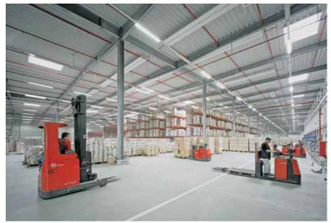
Zehnder ZIP radiant ceiling panels have shown themselves to have been a good choice: with extremely low convection and high energy efficiency, they represent the optimum solution in the 38,626 m<sup>2</sup> warehouse.
