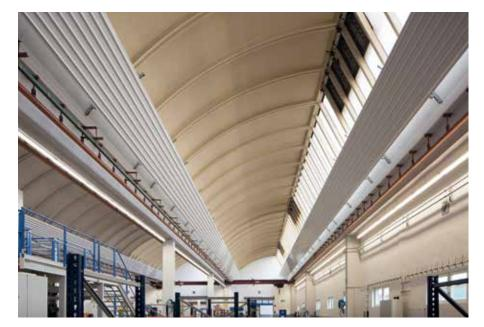
Flexible installation: in an older hall with a saw-tooth roof, it was no problem to suspend the Zehnder radiant ceiling panels parallel to the ceiling and adapted to the room geometry. The 20 per cent inclination does not compromise efficiency or how easy it is to distribute heat across the radiant panels.
