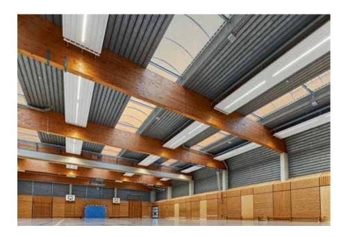
In the Georg Schindler sports hall, a total of 24 Zehnder ZBN radiant ceiling panels with recessed LED light fixtures were installed. The energy-saving 2-in-1 solution was mounted on wide span beams using chain suspension. The individual radiant ceiling panel elements were connected using flexible connectors, which were routed along the ceiling construction several times through glued laminated timber bores.
