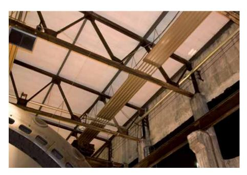
These were solved with Zehnder ZBN radiant ceiling panels with surfaces made of untreated steel. They blend inconspicuously with the general appearance of the site; therefore the view of the roofs of the steel construction is retained.
