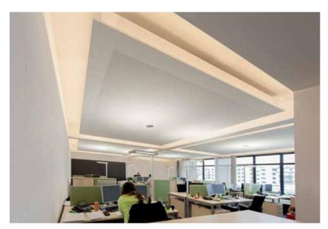
In contrast to conventional circulated-air cooling systems, Zehnder plasterboard sails use passive cooling involving cooling elements, which are easy to integrate in any ceiling at little expense and without compromising the appearance of the room.
