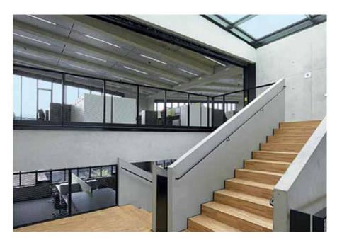
The "folded" roof on the top floor also poses no obstacle: the customised ceiling sails were suspended in accordance with the slope of the ceiling.
