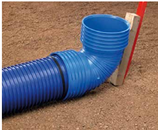
2. Use a wooden block to avoid damaging the elbow during assembly. Alternatively, use an iron bar or a spade.
