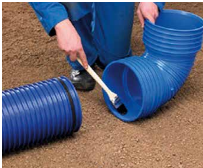
1. Fit the sealing ring in the second groove from the spigot end. Apply Uponor grease to both the sleeve and sealing ring.
