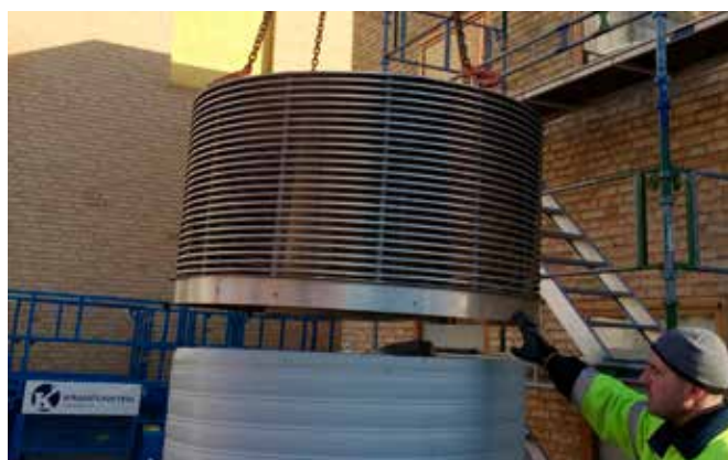
Attach the cap to the lifting lugs and lift it into place.
