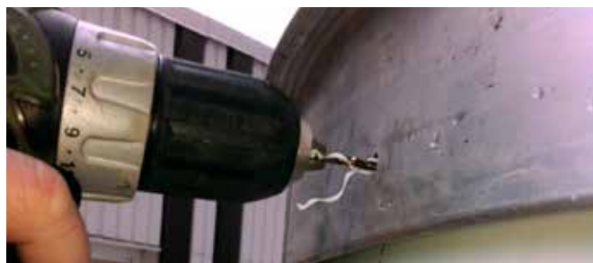
Pre-drill holes in the tower before attaching the tower cap.
