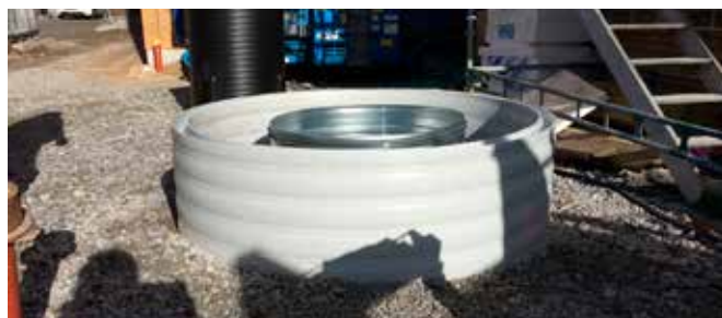
When installing the combination cap, make sure to connect the air outlet in the tower to the exhaust duct located in the middle of the cap.
